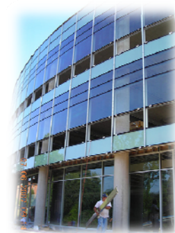
Curtain wall installation
